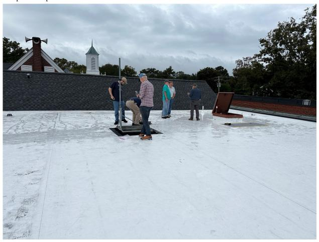
Club members returned two weeks later to finalize the installation. Pictured below the VHF/ UHF and HF end fed wire antennas are being terminated. An ICOM A4 remote tuner tunes the HF antenna from 80 to 10 meters. The weighted support pole is placed over the gym roof in close proximity to the hatch access located in the second floor storage room where an equipment cabinet houses the ICOM 7100, power supply, PC, router and remote control hardware.
